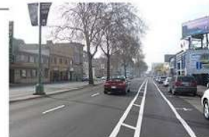
A street with two lanes in each direction and a center divider with a buffered bike lane
