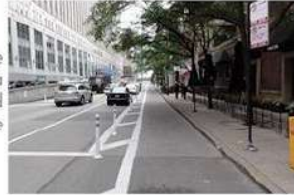
A four-lane street with a separated bike lane
