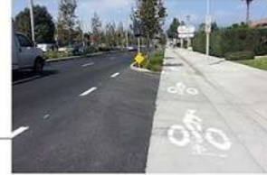
A street with two lanes in each direction and a center divider with a separated bike lane
